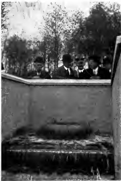
Discharge Chamber of Reservoir, at New Westminster.
